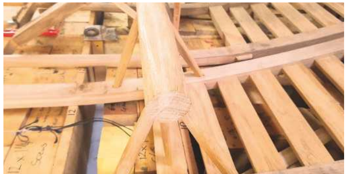
33 Cross post of front assembly
