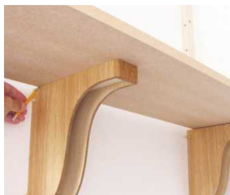
24 Cut 18mm MDF shelving to size and round off the front corners if necessary. Notch rear edges for the uprights
