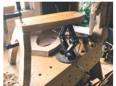
3 Installing the back legs – a car jack came in particularly handy here!
