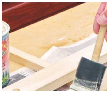
21 Lightly chamfer edges of uprights and finish with two coats of suitable paint to match the bracket
