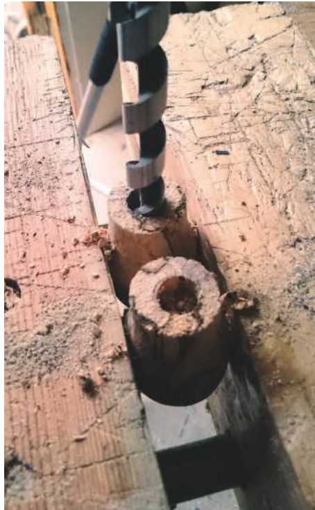
27 Drilling holes for the screws
