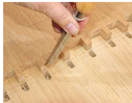
11 This row of mortise & tenons are cut with a standard dovetailing jig using a straight cutter. Round-ended sockets are quickly squared up with a mortising chisel
