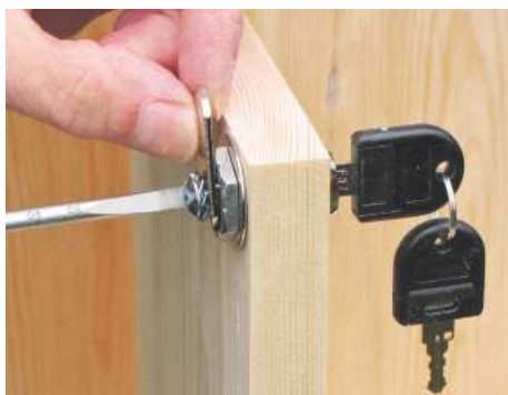
18 Drill a hole in the top corner of the door to suit the barrel of a cam lock. Insert and fit the cam lever to the rear
