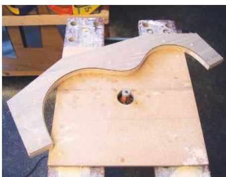
8 The hardened edge of the template attached to the mould board for final finishing
