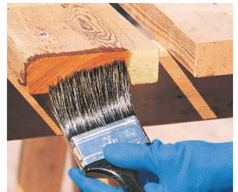
Applying preservative with a brush, ensuring the end-grain is especially well covered
