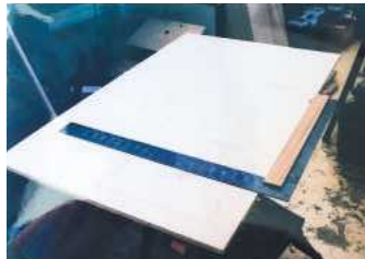
As Ray shows, the steel roofing square is a very useful setting out tool
