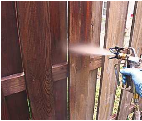
Applying preservative with a spraying system
