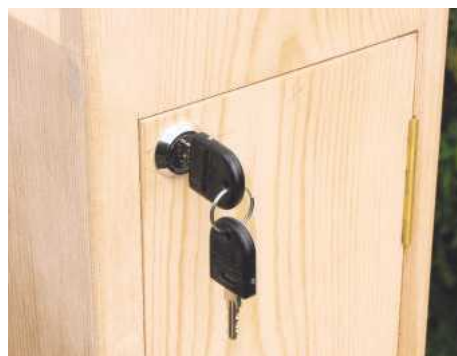
19 Check the door closes and the lock operates correctly. Make adjustments if necessary
