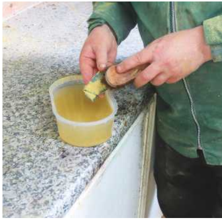
23 Clean the abrasive regularly with water
