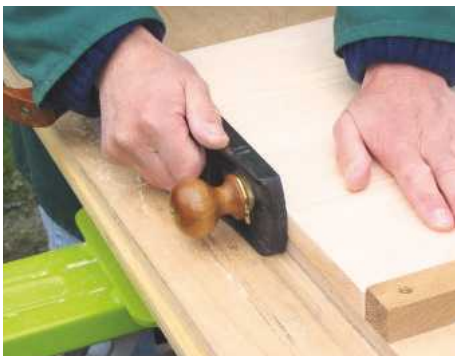
5 Saw all panels to size and plane ends square using a shooting board for accuracy
