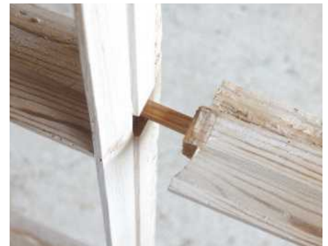
The actual profile was not quite an ovolo, more a slimmed down version to suit the narrow bars
