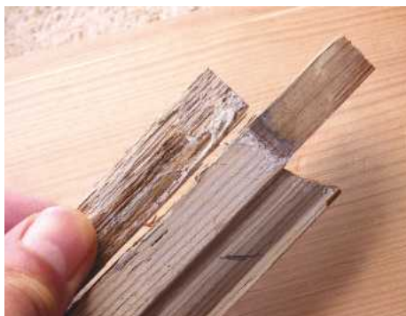
25 Some glazing bars are likely to split when removed from the bottom rail, though it's easy enough to glue these back together
