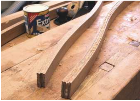
3 The glue squeezes out while the laminate sets to form beads around the edge (right). The laminated components are edge-planed as soon as the glue sets but before the resin becomes too hard (left)
