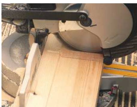
10 Cut the tenon shoulders on the bottom rail with a sliding mitre saw or bandsaw. Remove the waste material from the cheeks
