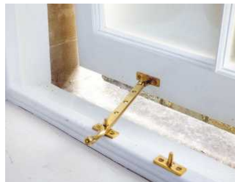
36 Fit a pair of traditional casement stays to each sash. If using brass screws, insert steel ones first to prevent damage to the slots
