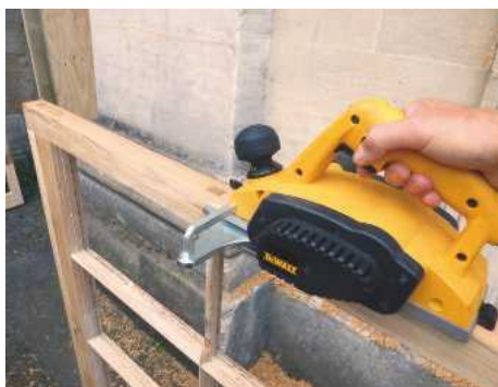
31 Both outer edges of each sash will need to be planed. This will create sufficient clearance for opening when fixed into the frames
