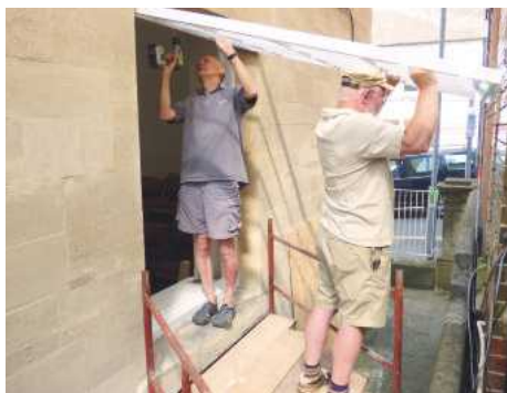
34 Three stainless steel hinges are used on each sash. Once removed, the sash can be finished with a suitable exterior paint system
