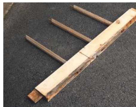
6 With the rail removed, number each glazing bar before dismantling. Saw through the rail alongside each bar if they're tight
