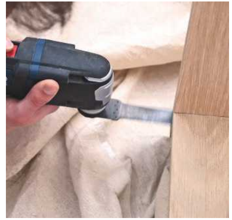
Cutting notches into a cabinet carcass
