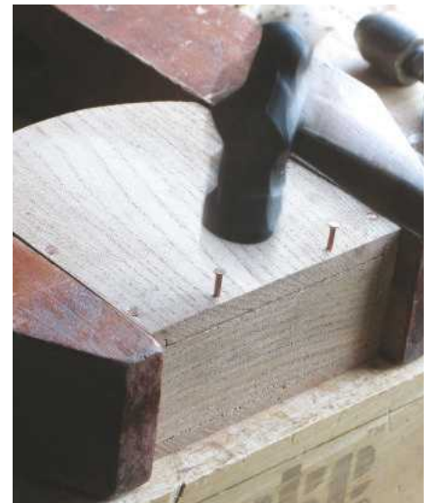
30 Strike the nail squarely to avoid a glancing blow
