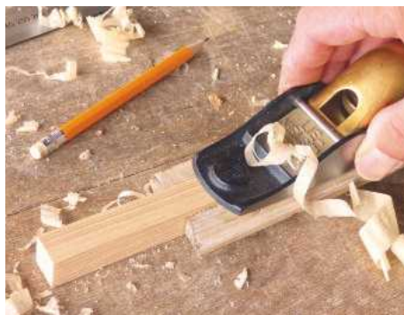
26 Other bars may need more in the way of repairs. Where necessary, cut away damaged wood and splice in replacement pieces
