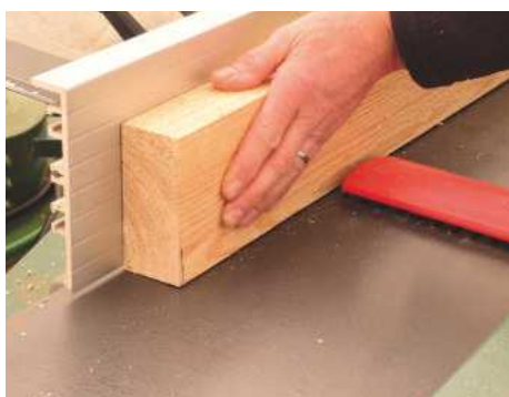
7 Plane new timber to size. Bottom rails and stiles finish at 45mm thick, though allow extra for final planing up when assembled
