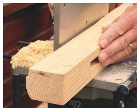
12 With a table-mounted router, machine a profile along the inner edge of both stiles and bottom rail. Do the same with the rebates
