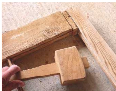
5 Tap the bottom rail away from the stiles, taking care not to damage the attached vertical glazing bars, which may work loose
