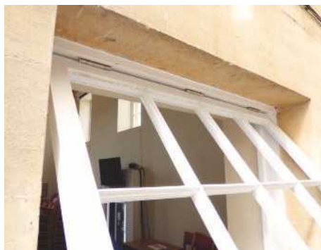
35 Refit the sash after painting and check it opens and closes without binding in the frame. Then it's ready for the replacement glass
