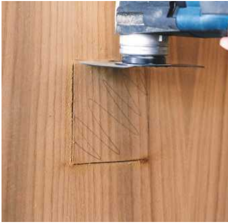
Cutting a slot for an electrical switch in MDF
