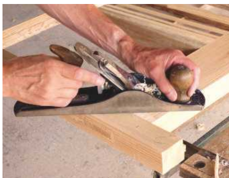
28 Once the new bottom rail and stiles have been glued to the sash, plug the screw holes and trim flush. True up surfaces with a plane
