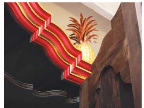
8 With the upper door open, you can just about make out the shaped frame behind the cornice
