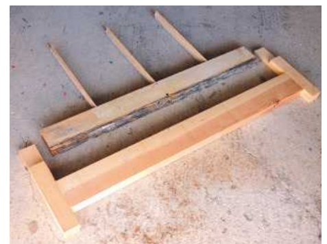
21 The replacement bottom rail is slightly wider than the original one. This enables a bevel to be sawn after gluing everything together
