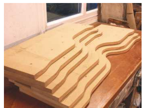
11 MDF running boards for cornice
