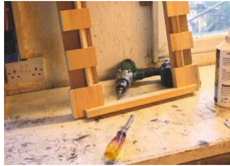
8 Fitted threshold, tying together the base of the mirror surround
