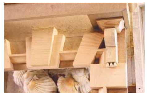
20 Guttae glued in place – the surround is now ready for painting
