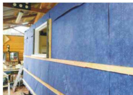
Some 25mm batten work now in place over the membrane
