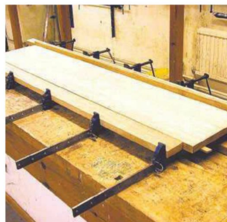
6 ... ready for the front lippings, which will need to be cramped in place with a timber batten, or...
