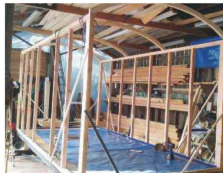
Studwork frame of 2 x 2 and 4 x 2 Douglas fir glued and screwed with diagonal braces
