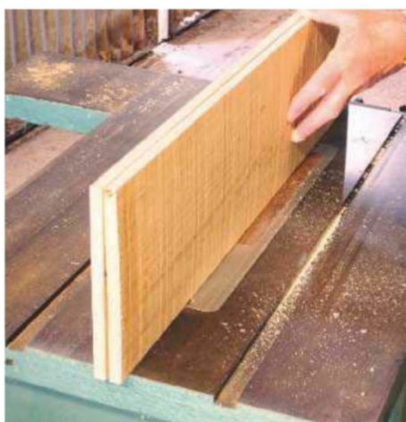
14 The shelf is deep cut against the fence (not visible)
