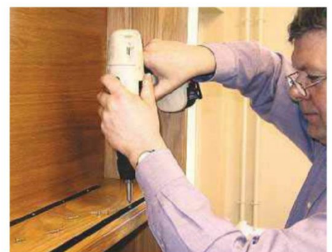
19 Finally, fit the shelf tracks, ensuring that all the slots in each set of four line up perfectly
