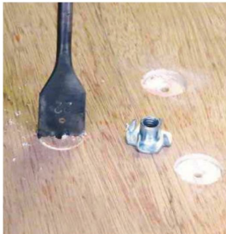
6 ... and countersink so that they sit flush to the ply
