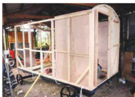
The inside of the hut is lined with high quality plywood to give stability and strength
