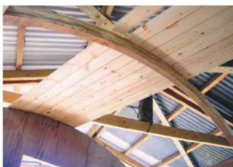
The ceiling is laid with tongue & groove boards onto the curved beams
