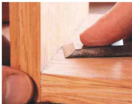
3 Scribing width with a chisel for the first corner rebate...
