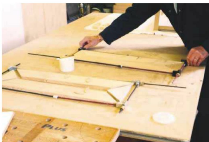
22 The top pad frames are glued and clamped up
