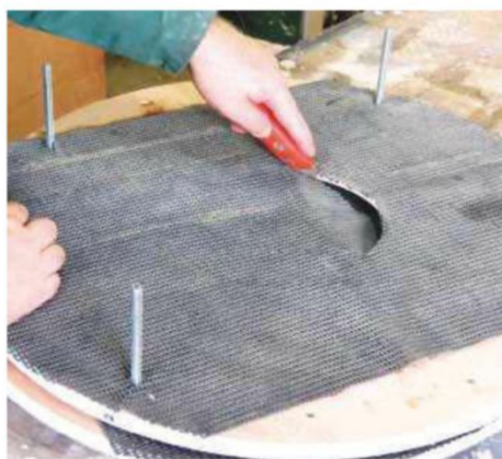
12 Stick non-slip router mat to the inside surfaces of both discs
