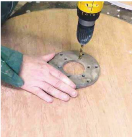
5 Mark the location for the 'T' nuts...
