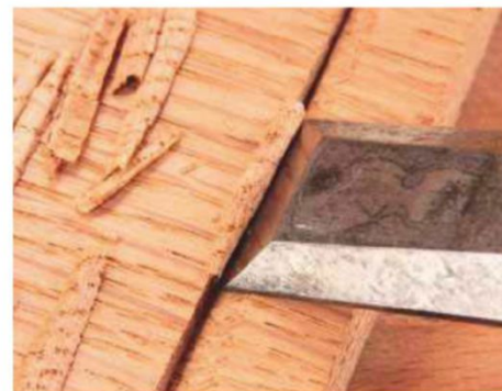
7 ... before chiselling out a trench and shoulder...
