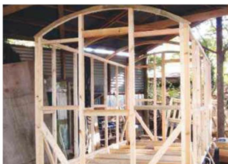
The framework attached to the chassis. The chassis is two axle assemblies linked by a pair of longitudinal angle irons
