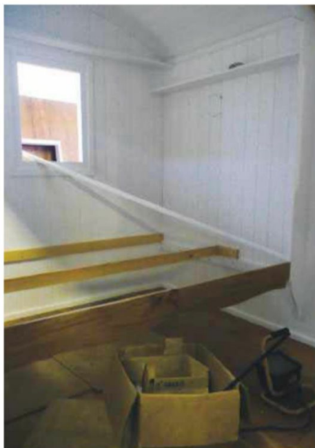
Oak floor bed construction in progress
