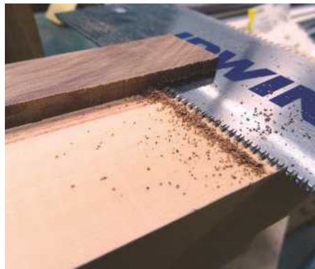
15 Sawing the ends of the rails flush with the edges of the seat
