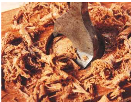
18 Boring a 25mm hole for the peg
