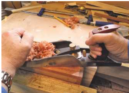
11 After glue-up, the box is cleaned up and the front flushed down to the ends
