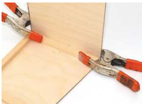
8 Glue the sides to the bottom piece and then proceed to clamp up
