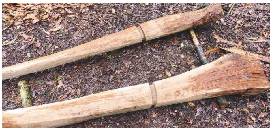
A couple of posts showing their seat grooves
