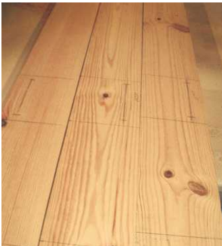
1 After taking care to orient the posts, the mortises were marked out to one side
