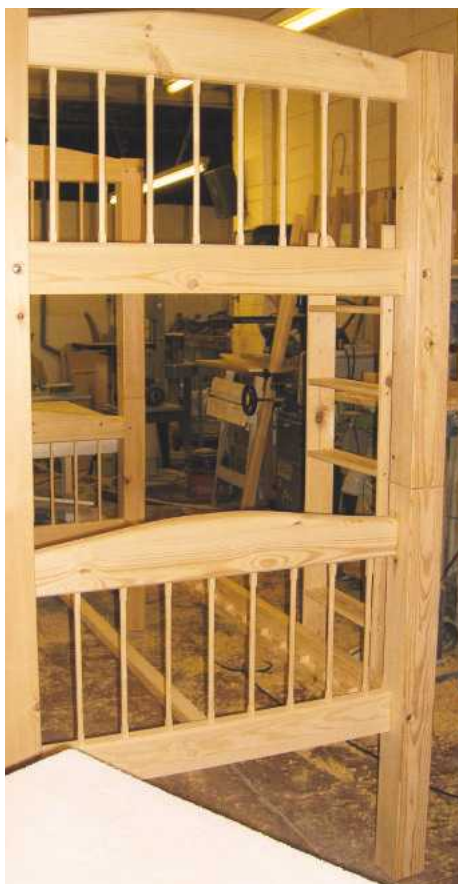
19 The centre rails were mortised into the boards with loose mortise & tenons
