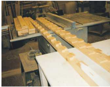
26 Bearers were cut on the radial arm saw ready for fitting to the pull-out frame
