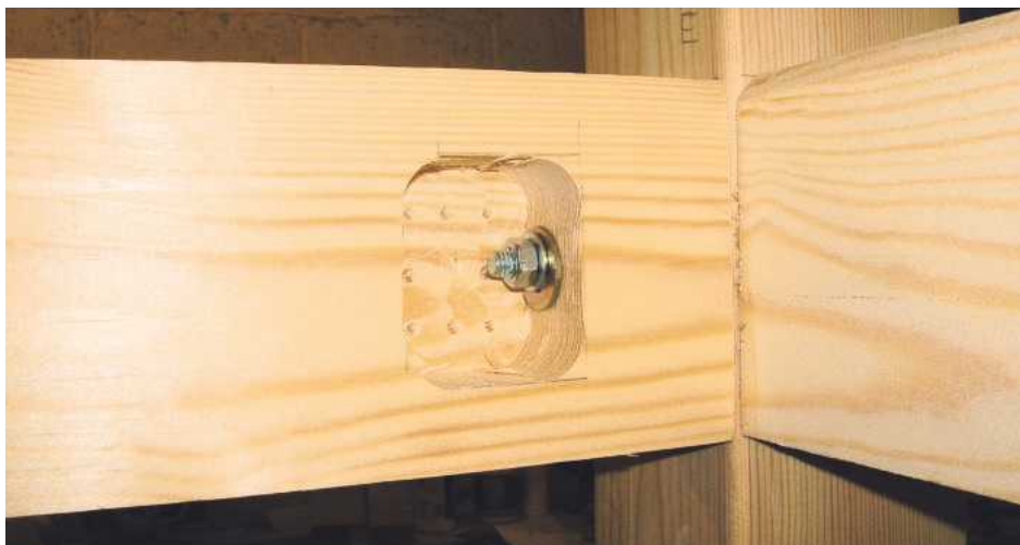
16 The next job was to drill and test fit the rails
