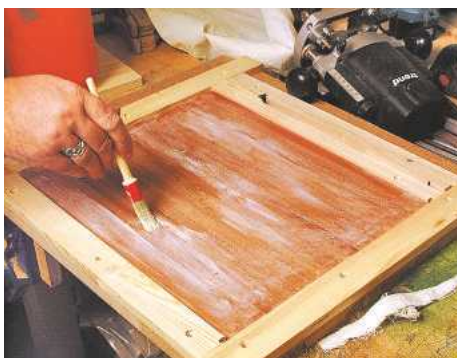
13 Use the jig to hold the slats tight together as you glue them; try not to let glue run down into the joints
