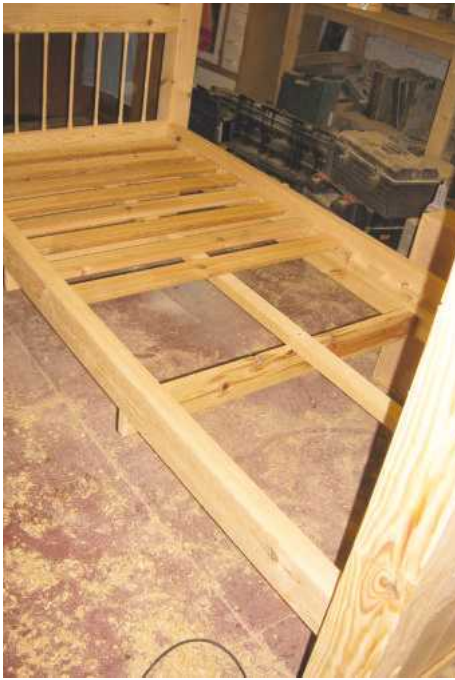
22 The drawer frame that hangs below the lower bunk was fitted in place below the bottom rails
