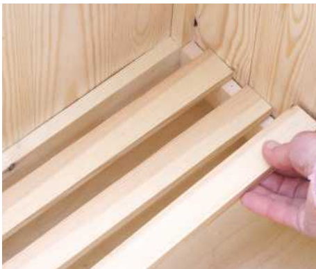
14 Cut slats to length from the door stop. Either pin these to the lower rails or use a nail gun
