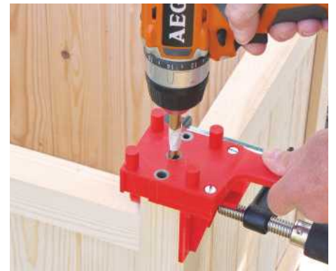
16 Cramp the dowelling jig in position and drill each stile with a 10mm lip and spur bit
