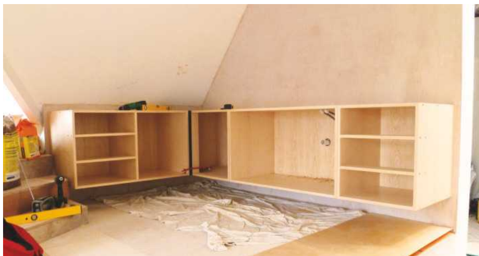
12 Fitting the cabinets to the wall
