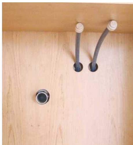
11 Pipework fitted into one of the cabinets
