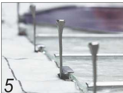
... and holding everything in place with flat-sided horseshoe nails tapped into the lead board
