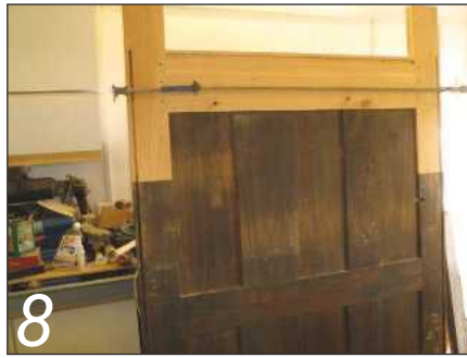
Back complete with spliced stiles and bottom rail
