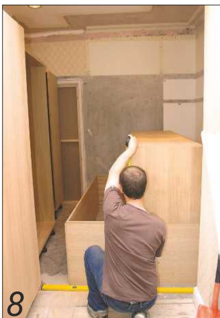
Assembling the carcasses in the workshop prior to installation made for a much easier site visit. Note adjustable feet for convenience
