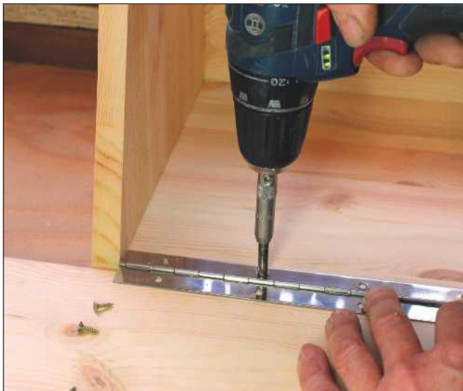
Fixing the hinge in place, the use of a centre pilot drill bit makes this job virtually fool-proof
