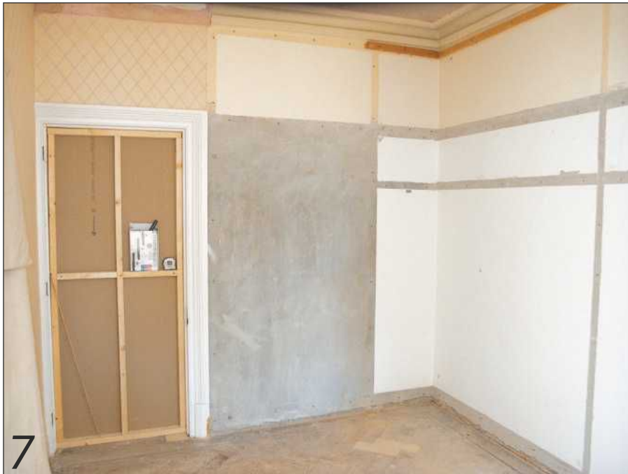
I decided that an L-shaped suite extending from floor to ceiling and running along two walls was the most efficient way to construct the wardrobes in terms of space
