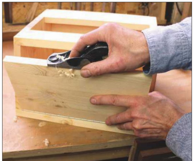
Planing the leading edge of the door to a nice tight fit
