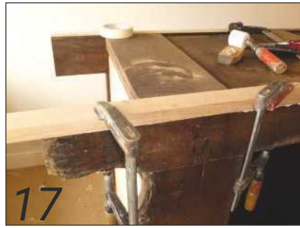
17 Splice glued in place
