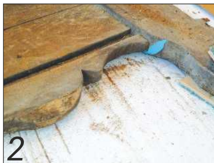
2 Section of waney-edge on the inner apron
