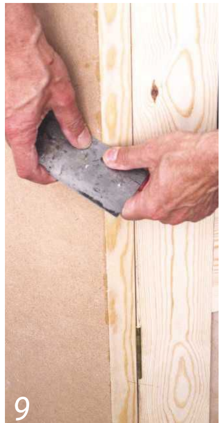
9 Cleaning up the carcass corners on site; a scraper really is an invaluable tool
