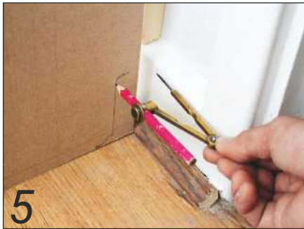
5 Scribe the sides into the wall and skirting board before cutting with a jigsaw
