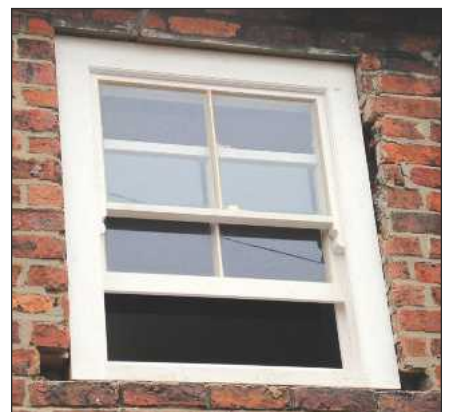
Mould the parting and staff bead; cut and fit the parting beads with the outer sash
