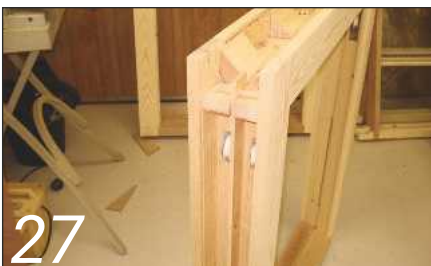
The final move is to hang the wagtail in place and slide in the 6mm ply back
