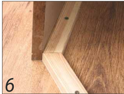
6 The sides are checked, then glued and pinned into place. Note matching bevel on front edge
