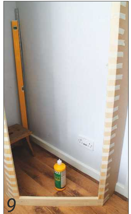
9 After any necessary adjustment, the frame is put together and glued into place
