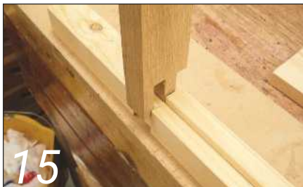
15 Mortise & tenons joint the sashes, only the joint between the rails and stiles differing
