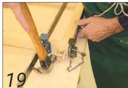
19 Vertical glazing bars should always run the full height of the sash and be through tenoned and wedged at meeting rails
