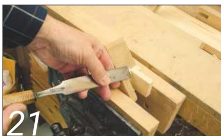
21 The outer faces will need the mouldings mitred at the top corners and cut out to sit on the sill
