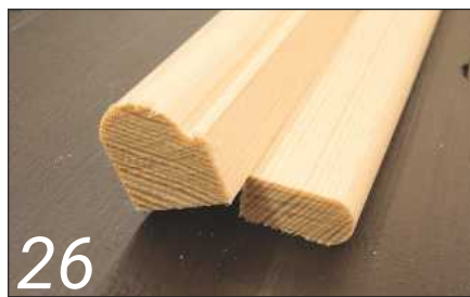
Mould the parting and staff bead; cut and fit the parting beads with the outer sash
