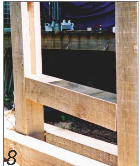
8 As it's a loose fit, the sliding beam can be fitted at an angle after fixing the other timbers
