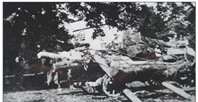
Unloading was a skilled job in itself
