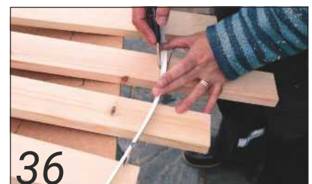
36 Mark out the curve on the back using a suitable lath
