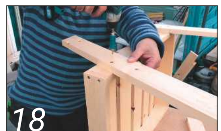
18 Align each leg to the layout marks and screw in place
