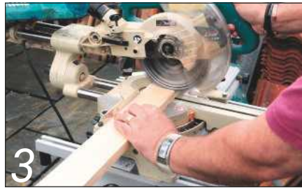
3 Cut the seat slats, front and rear seat frame components at 450mm long
