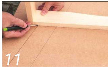
11 The seat frame is positioned on the rod to transfer the leg splay positions
