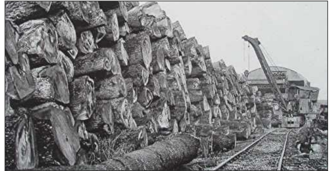
A mobile steam crane on rails was necessary for the huge amount of timber requiring processing
