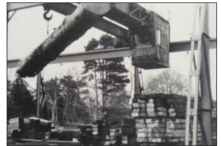
The gantry crane in use for sawn and unsawn timber
