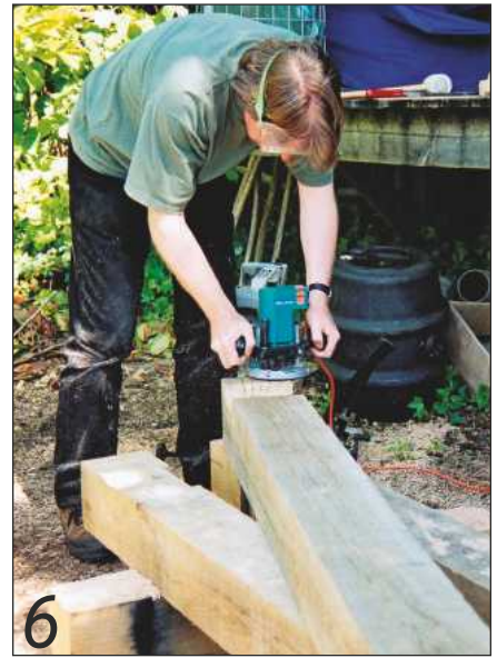
6 The timber arrises of the posts and lower beams can be cleaned up with a router
