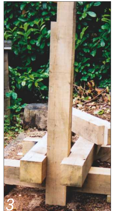
3 Cut checks at either end of each beam to make a tight fit with the posts
