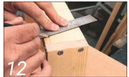
12 The marks are connected to ensure the legs are positioned accurately when fixed
