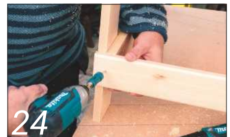
24 You can then round over the edges and screw into place
