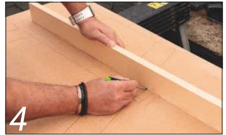
4 The rod is now used to transfer length and layout positions for the sides of the seat frame
