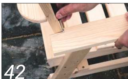
42 The initial cut will need scribing to allow for the angle of the back slat
