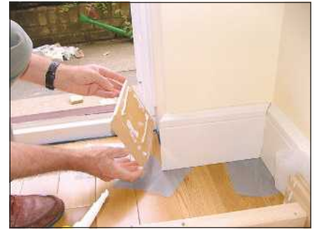
...you may need to bend the skirting to shape if the wall is uneven
