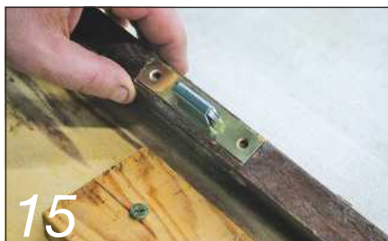
15 Installing a new lock to the lift rail
