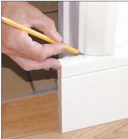
Fitting the skirting below a vertical architrave...
