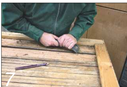
7 I used a paint scraper to give the slats a final clean up until...
