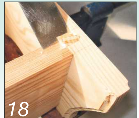
18 Trimming a corner of the rebate with a chisel
