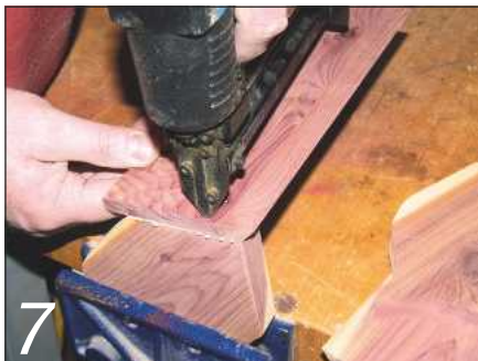
7 Nail the first roof segment in place, aligning it with the rear edge of the back panel
