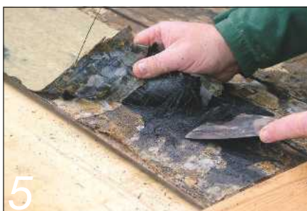
5 A wallpaper scraper could remove some of the perished backing...
