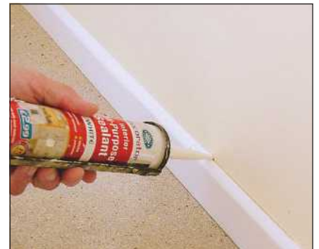
Apply a polymer sealant to make an effective and neat seal
