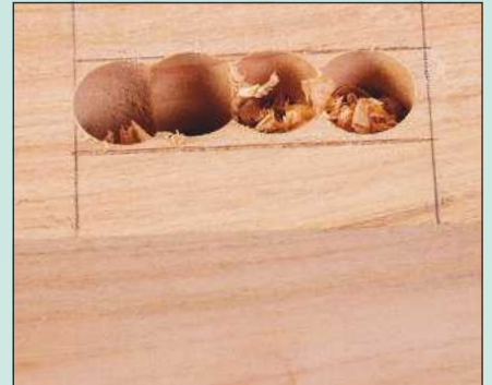
7 The majority of the waste is now removed ready for cleaning up
