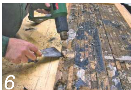
6 ...but other areas needed a heat gun to loosen the glue
