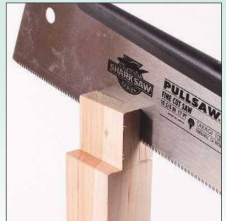
10 Stand the rail up vertically in a vice and cut down the tenon cheeks
