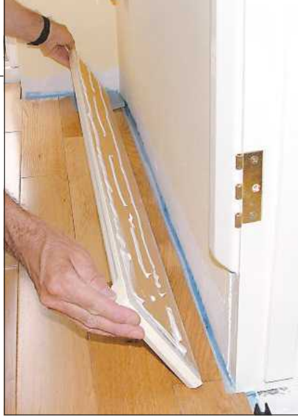
Continue working around the walls, remembering that...
