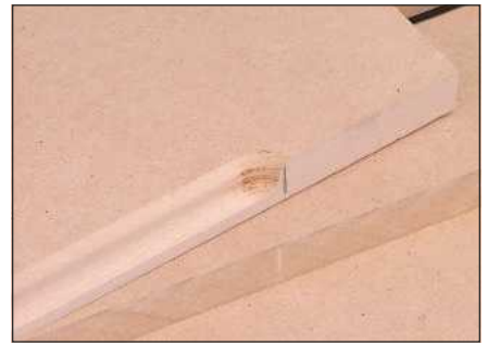
This moulding was stopped short so that it could be run underneath a door architrave
