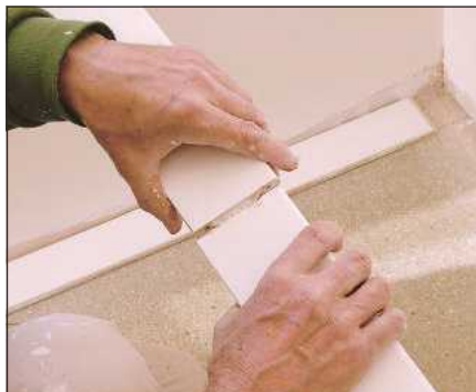
For long runs, join the skirting with biscuits and adhesive
