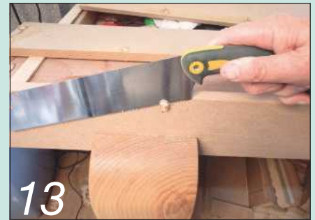
13 ... before being cut off flush
