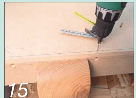
15 The screw holes were positioned central to the dowels, giving the screws a much better grip than in MDF
