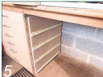
5 ... before screwing them in place in the cupboard space
