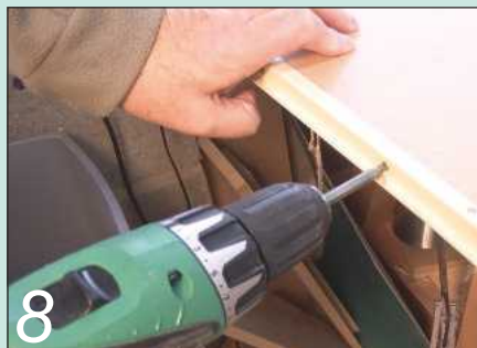
With the shelf inverted, bottom-mounted runners were fitted, offering good support
