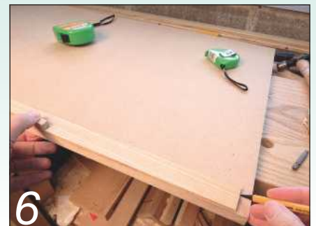
6 I measured the internal space precisely using overlapping rods
