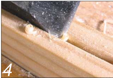
4 Easing the corners of the slot with a chisel makes the guard easier to fit
