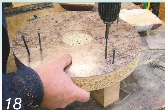
... and then screw them more securely through the back of the ply
