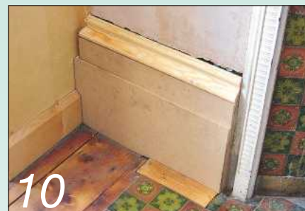
10 The new skirting is built up using MDF and the new top moulding
