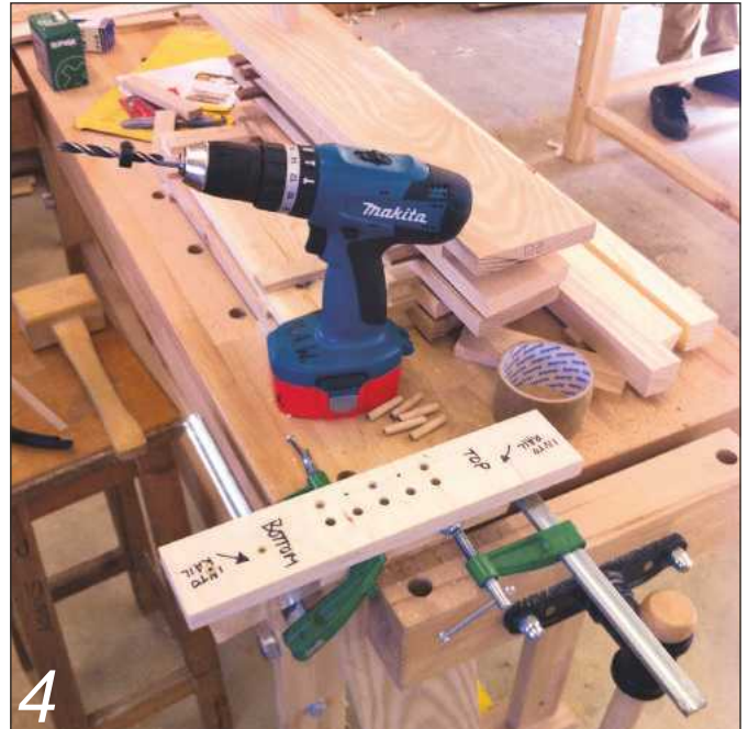
4 Precision drilling is required to ensure the rail bolts and threaded inserts will always line up
