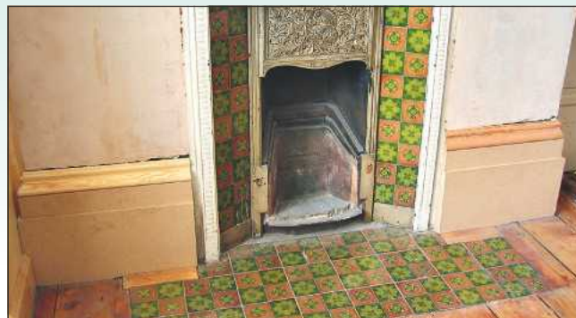
10 The new skirting is built up using MDF and the new top moulding
