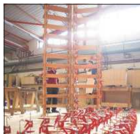
The first two sides go up and the structure starts to take shape, thanks to a veritable forest of cramps
