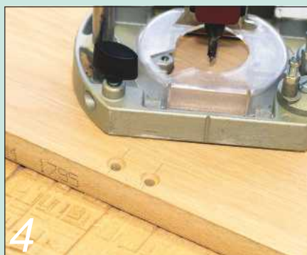
4 Bore holes in the top and base for the screws that will pull the housing and rebate joints tight
