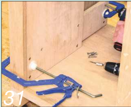
31 To set the correct runner spacing, mount the runners on spacers made from plywood
