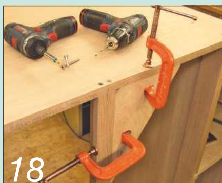
18 Prepare and attach the back jointing strip to the base and top. Plywood webs ensure squareness
