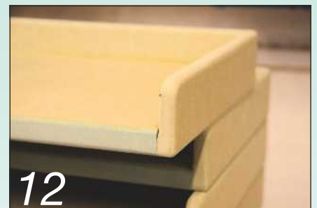
12 ...you can see there's a gap in the joint at the front which will need filling later
