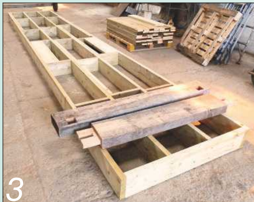
3 Having such a large flat work space in the barn was a real blessing as we assembled the deck frame
