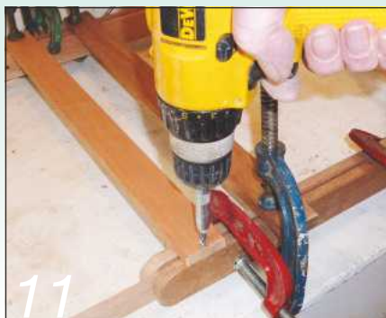
11 Drill holes for the fixing screws in the cross rail of the leg frame
