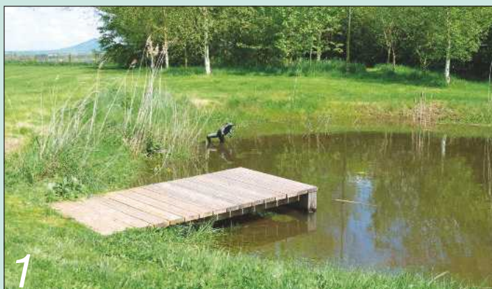
Our own small jetty has an oak frame and joists below water level, with a treated softwood deck resting on top of it
