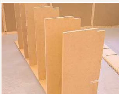
I decided to fit all the shelves to one of the side panels first...
