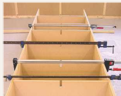
I squared up the carcass, cramped it securely and checked that it was all square
