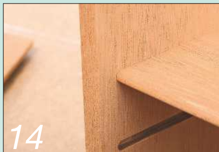
14 The resulting fit in the routed grooves was very neat and visually pleasing
