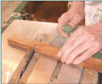
1 Cut angled ends on the top bearers. The saw guard has been removed here for clarity
