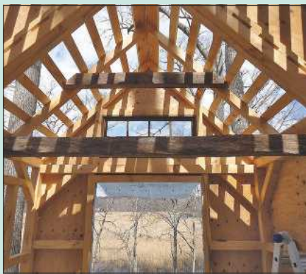
The main framework featured a mixture of old and new timber
