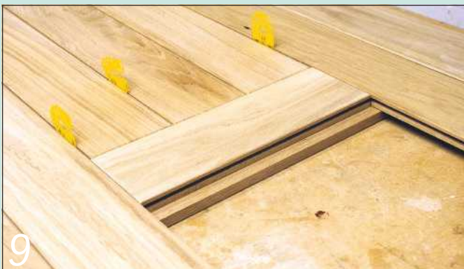
9 The outer section of the centre rail is tongued and grooved all round
