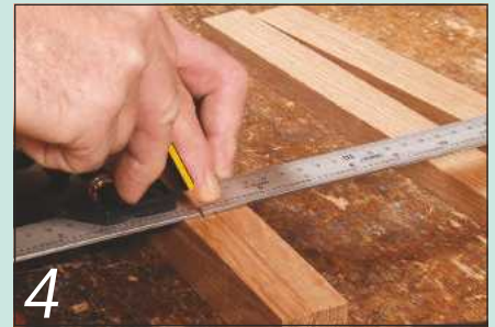
4 Mark the mortise positions with a sharp pencil; a knife cut will show on the finished piece
