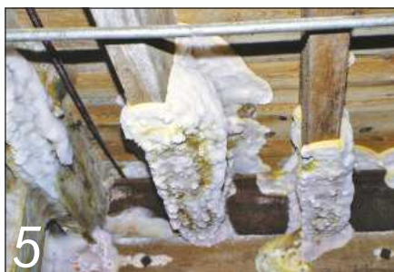
The most dangerous fungi of all, such as the dreaded dry rot, attack wood while it's in service
