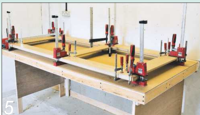
5 It was now time to glue up the external frame using plenty of cramps
