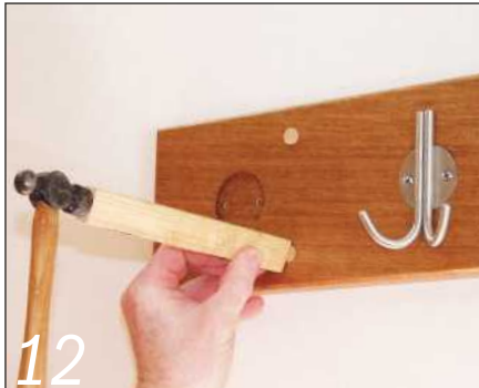
12 Counterbore the holes for the wall fixing screws and tap in matching oak plugs
