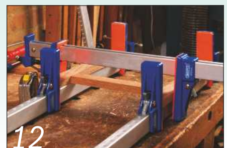
12 Glue and cramp up the frame components and check that the frame is perfectly square
