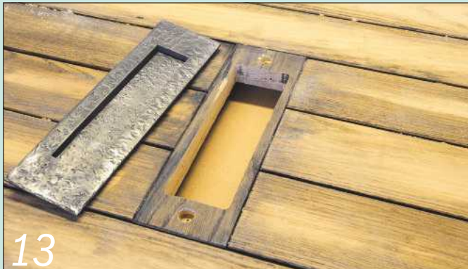
Test-fit the letterbox to check that it doesn't bind within its opening
