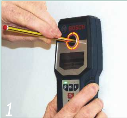
1 I used a hand-held detector to find the centre line of the wall studs
