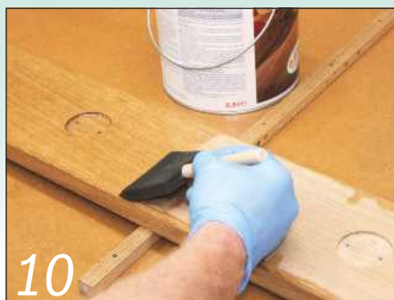
10 Chamfer all the edges of the back board and apply your chosen finish
