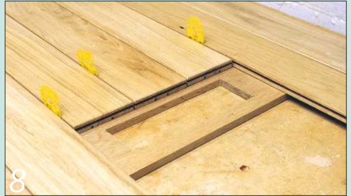
8 The outer boards run full length; the middle three overlap the centre rail
