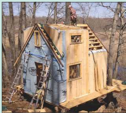
The external walls were soon skinned with insulation and cladding
