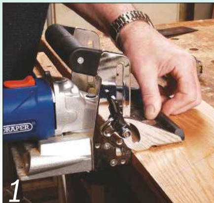
1 Cut slots for a couple of biscuits in each meeting edge to assist their alignment
