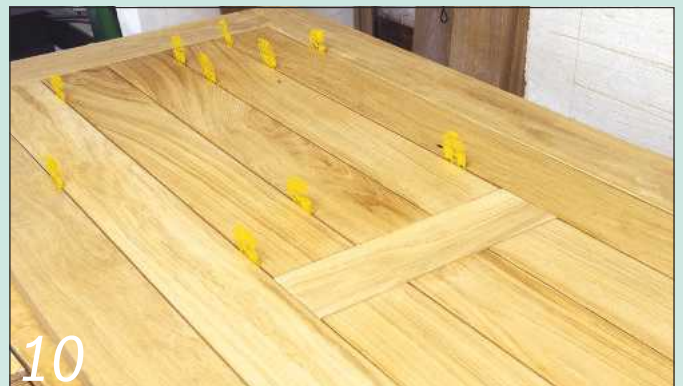
10 Complete the dry assembly of all the boards and check their fit
