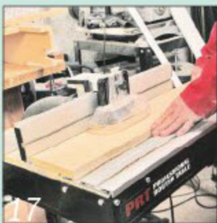
17 I cut a small chamfer on the skirting boards using my router table
