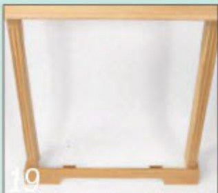
19 Pin small plywood offcuts to the batten behind the skirting board to support the front panel
