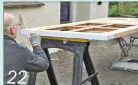
Cut the new door to size and hang it. Then remove it and paint the top and bottom edges
