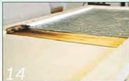
14 This left a smooth flat face, flush with the glass and the lower panel
