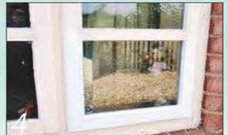
With the new glazing beads fitted and primed, the casement is ready for repainting
