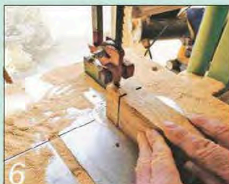
6 Cut the tenon shoulders on the saw bench and bandsaw the cheeks
