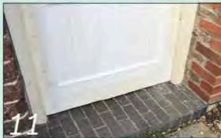
11 The repaired sections were replaced in the door and any gaps were filled
