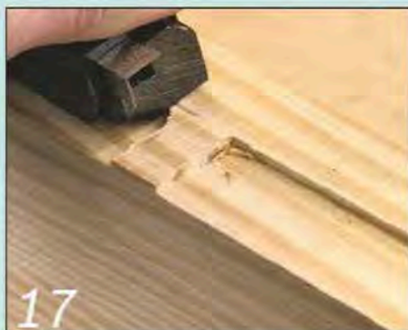
17 Tap the corner chisel sharply in each corner, then clean out the waste
