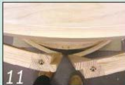
11 This door detail shows the inset catches, the scratch bead and the rebates (and my feet!)
