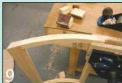
9 Cleaning up the curved door frames was a very satisfying process
