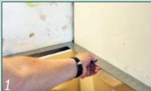
1 Carry out preliminary checks to see if the cabinets are square to the wall
