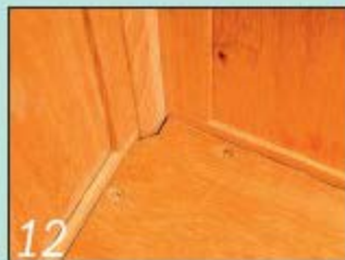
12 The plywood sub-floor is trimmed at the corners and then screwed to the support battens
