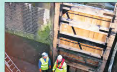
Once fitted, both gates need shooting in to ensure a watertight closure
