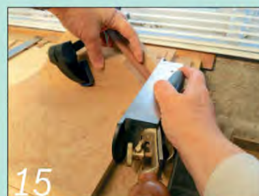
15 Cut the linings square, apply their finish and then mitre their ends using a simple jig
