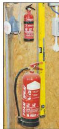
A foam extinguisher is best for oil fires, but is awkward to use
