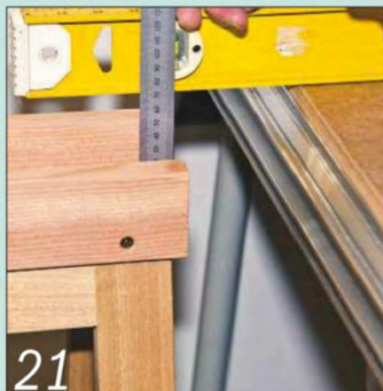
Check the finished height so you can calculate the size of the sacrificial insert accurately
