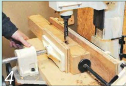
4 The bench mortiser makes light work of cutting the mortise slots
