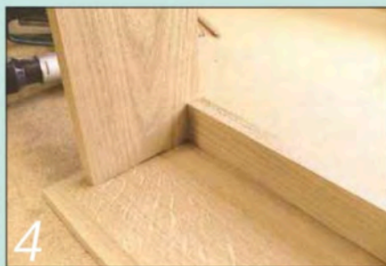
4 A dry assembly allowed me to check the fit and cut the two cleats accurately to length
