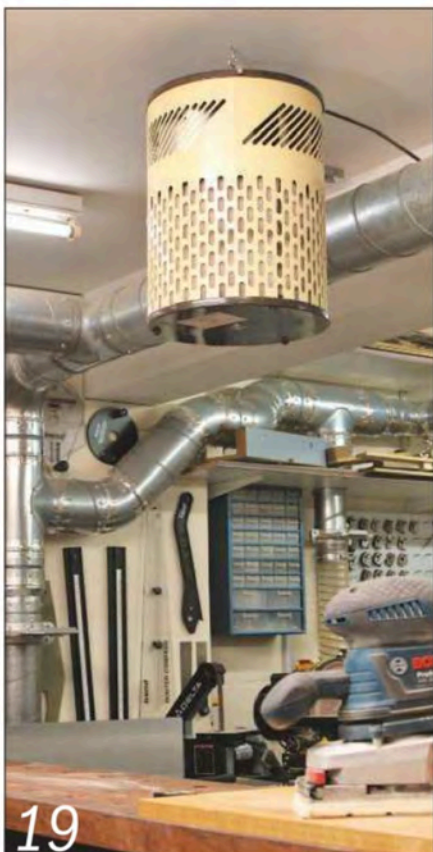
This old air cleaner is mounted above the bench and collects lots of dust
