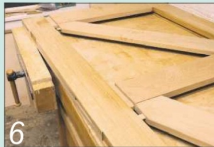
We removed the old mortises, made new rails and added a pair of diagonal braces
