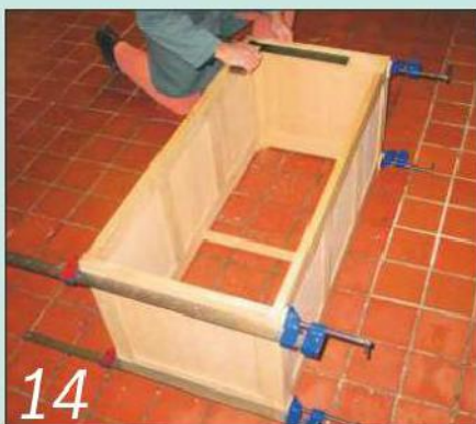
14 Complete the chest carcass by fitting the end rails and panels in place
