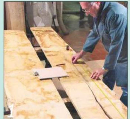
When marking out the various components, take care to avoid knots and splits
