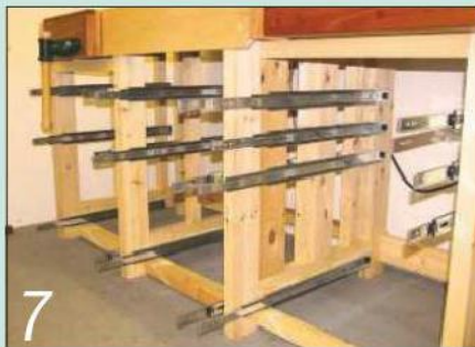
7 With the screw holes drilled, it was a simple job to fit the runners in place, ready to receive their tailor-made drawers
