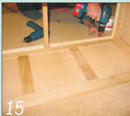
15 Screw and glue softwood battens to the lower rails to support the base panel
