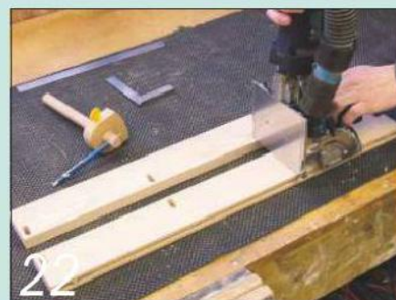
22 Cut the mortises in the frame stiles to accept the front and back rails
