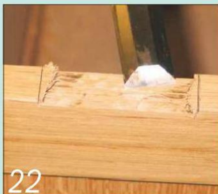
22 Chop out the waste from each hinge recess using a sharp chisel
