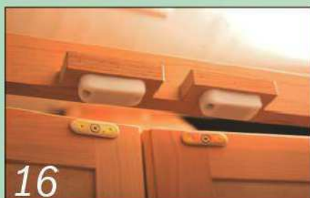
Add the magnetic door catches to the face frame on small blocks, and fit the keepers to the doors
