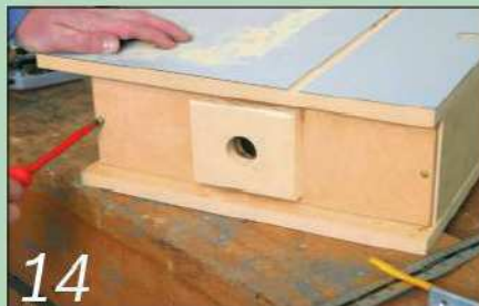
14 Fit a support boss for an extractor nozzle in the removable side panel
