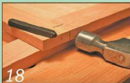
Unscrew each door and number it and its recess so you reassemble things in the right order
