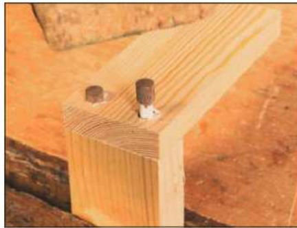
6 Apply glue to each dowel and tap it into place with a mallet
