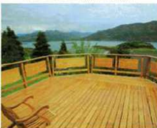
Decking - Construction in Larch
