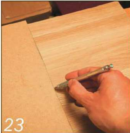
23 An mdf template ensured that the oak shelf was marked out accurately to fit the alcove
