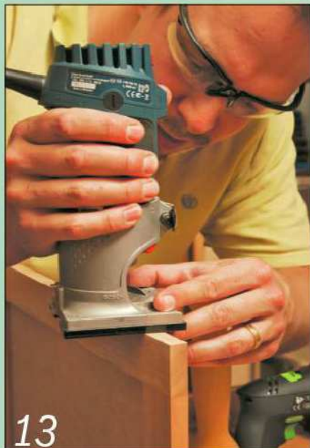
Mark out the hinge recesses and remove the waste with a palm router
