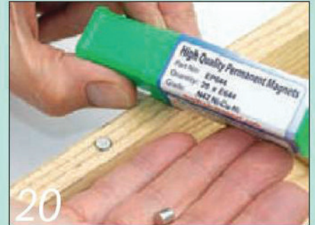
20 Bore a 6mm diameter hole 6mm deep into the carcass, and a matching hole into the inner face of the door frame. Glue small round magnets into the holes to keep the cupboard shut
