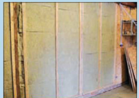
Rockwool slab insulation tightly fitted between the studs for improved sound insulation
