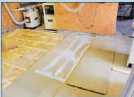
The flooring is two layers of 22mm chipboard. I staggered the joints and glued the two layers together with PVA
