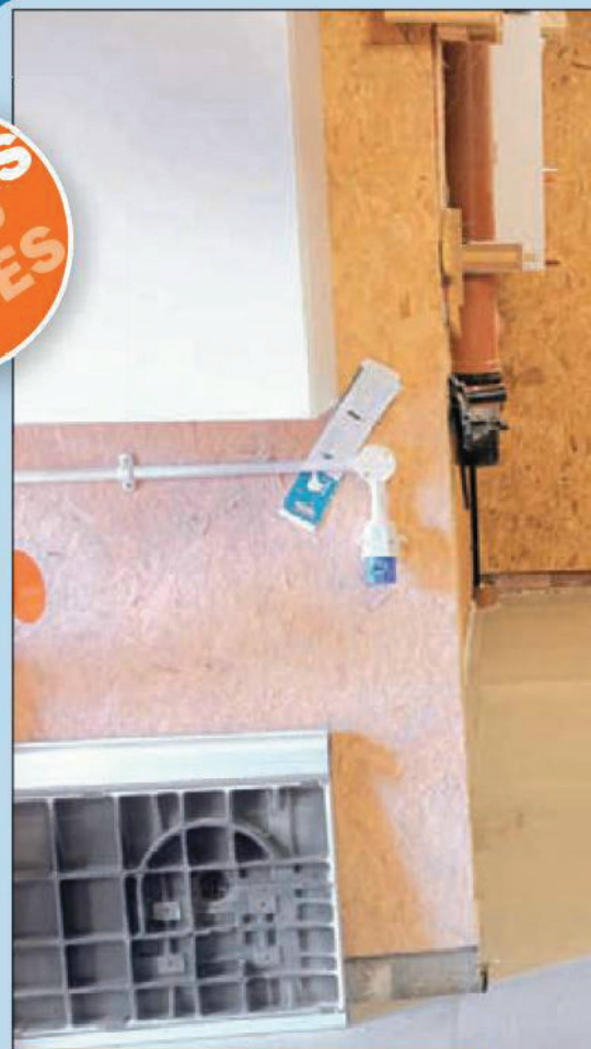
The finished floor is a vast improvement over the previous concrete floor. Now for some skirting boards...
