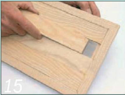
15 Trim the four panels to fit into the rebates on the inside of the door frame and glue them in position one by one
