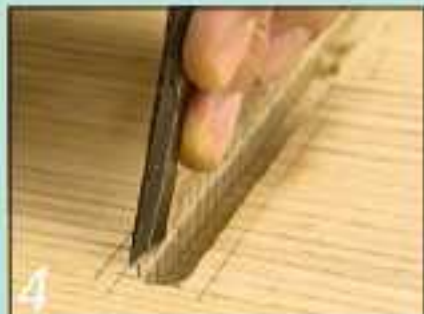
4 Squaring off the stopped housings with a bevel edge chisel
