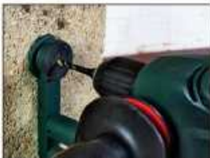
Drilling concrete with the dust extractor in place
