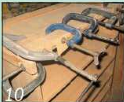
10 Battens support the base moulding while it is glued and cramped in position
