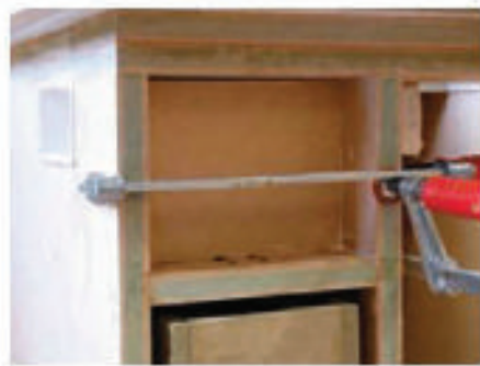
2 Two small pieces of MDF create the recess for the NVR switch
