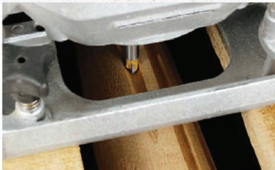
10 Start the cut in the middle of the flute, gently lowering the router as you move it forward
