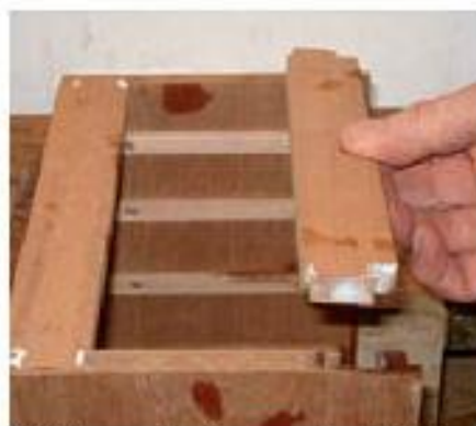
10 Start assembling the carcass by gluing the top rails into place
