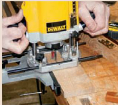
8 Cut the recess for the other flap. In this case it has to be cut a little way in from the edge of the timber, and therefore the fence has to be adjusted to suit this. Ideally the cutter should be the same width as the flap including the knuckle; otherwise the fence will have to be adjusted each time
