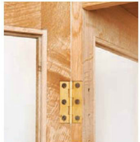
15 Hang the door, fit the catches and add a door knob to complete the cabinet
