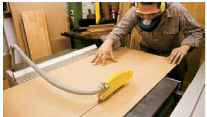
1 Cut the baseboard from a half-width sheet of MDF
