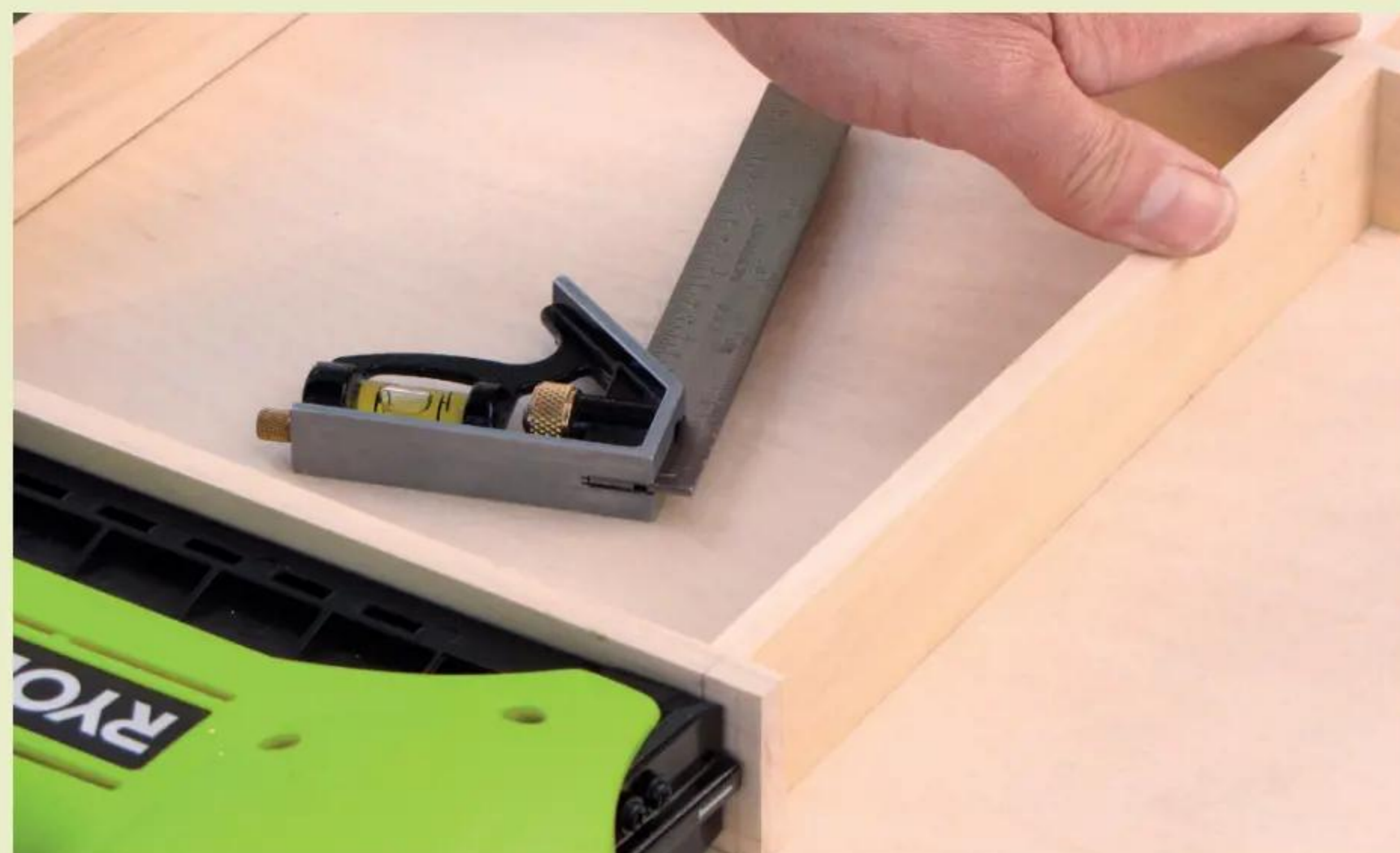
2 Glue the ends of rails and nail the framework together, checking geometry with a square
