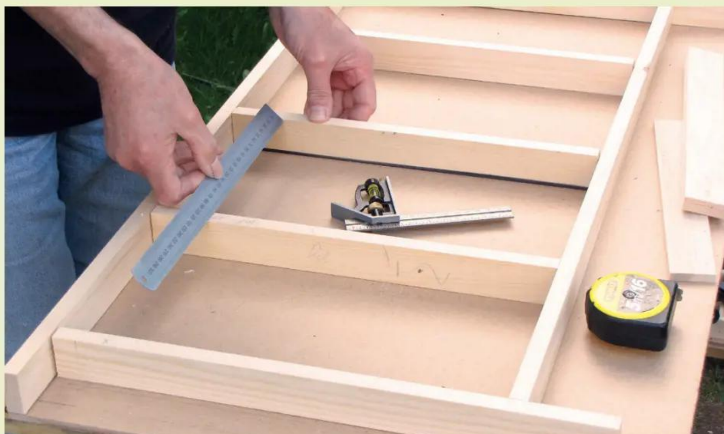
1 Decide on the layout of framework cross-pieces. These are spaced about 200mm apart
