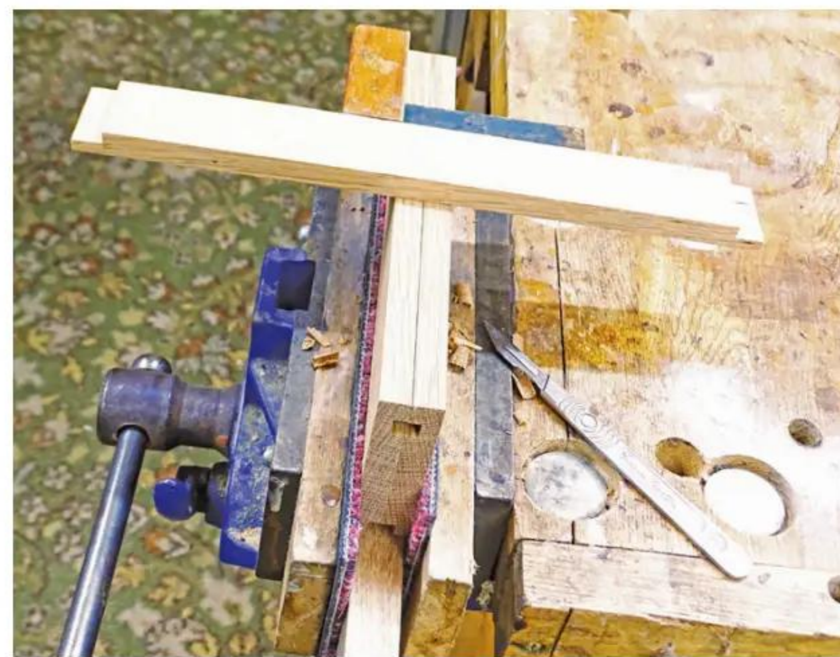
6 Ensure the timber is held at right angles
