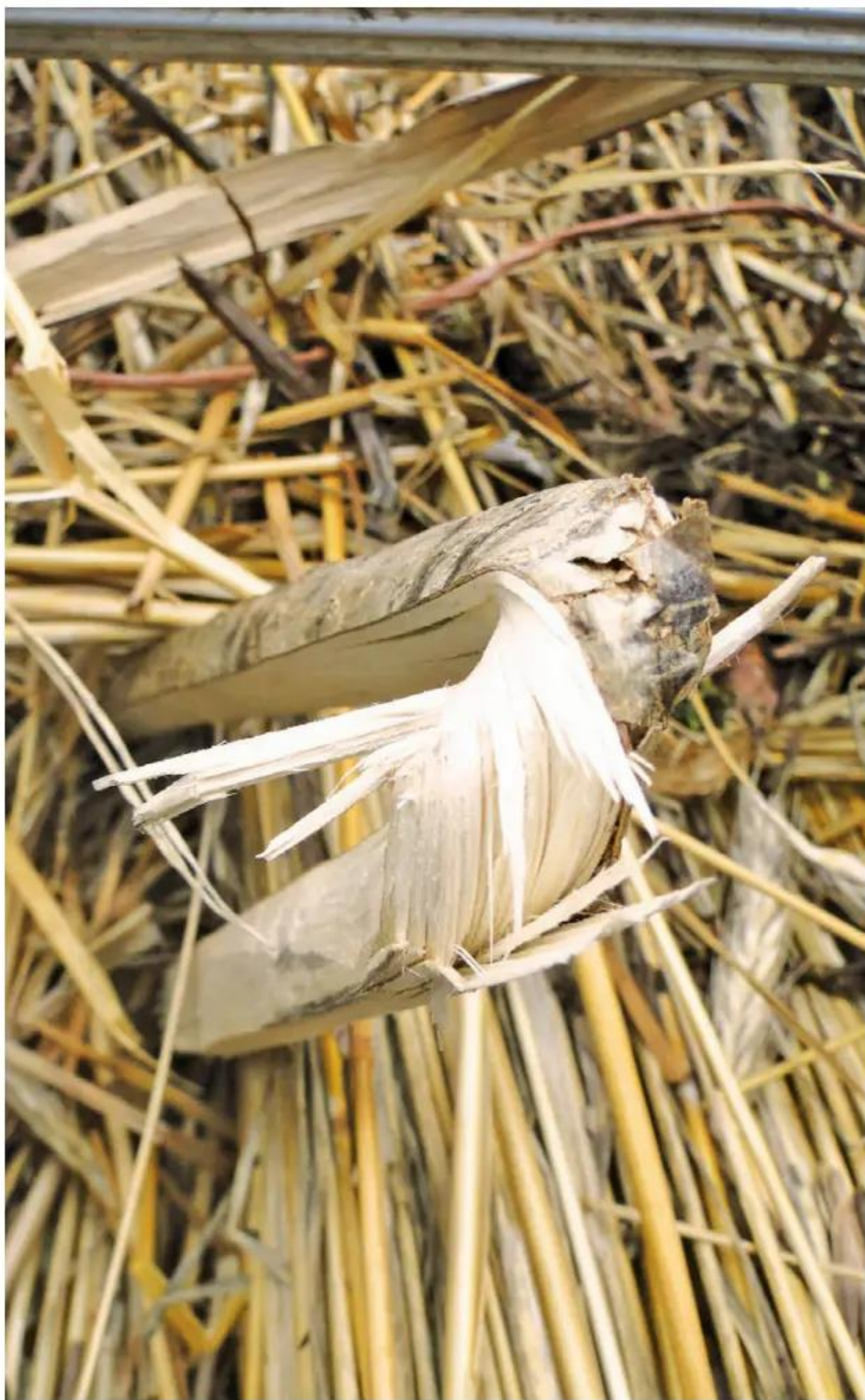
The straw and reed are laid on carpenter-installed roof timbers
