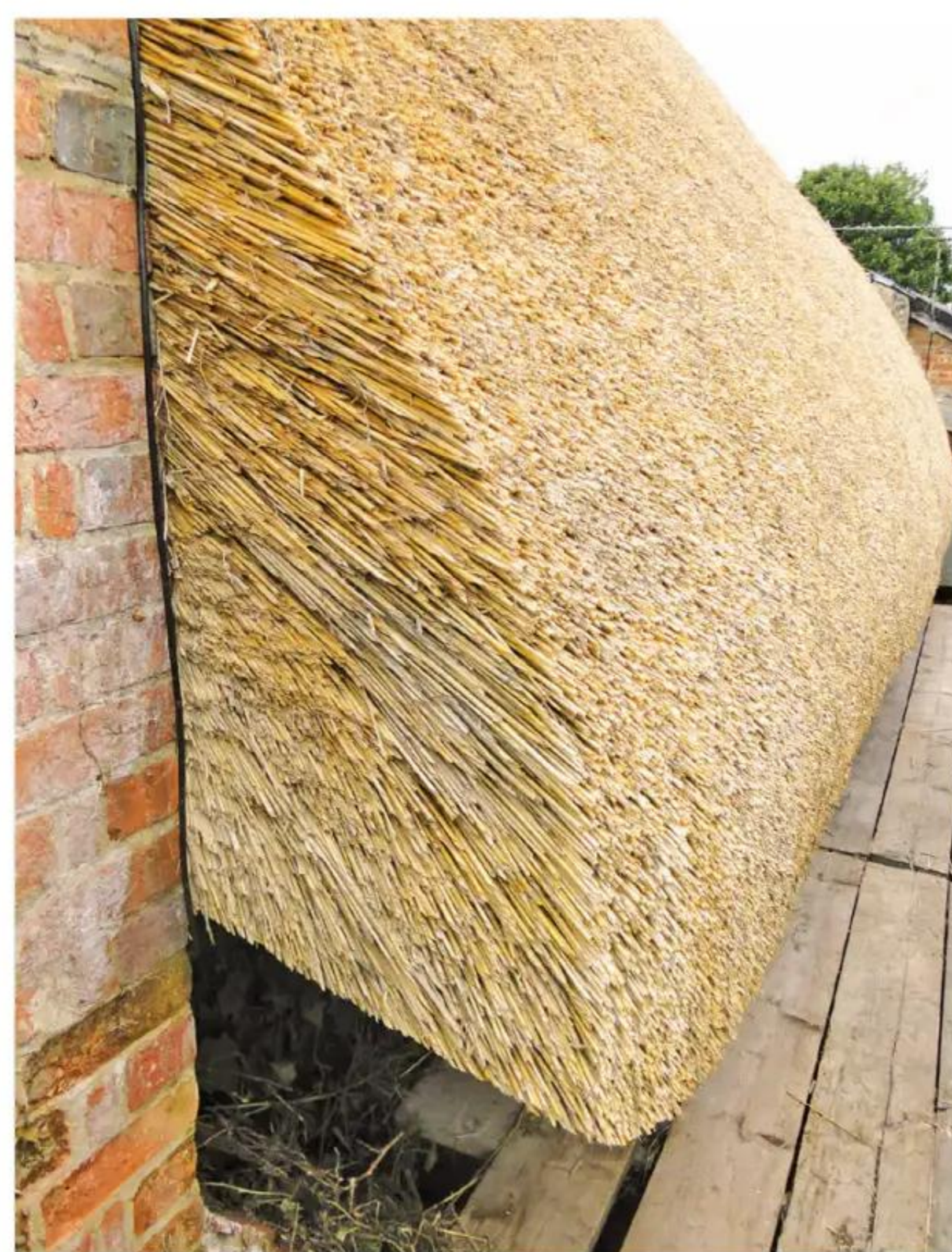
The Hewletts work with long straw, combed wheat straw, water reed and Norfolk reed
