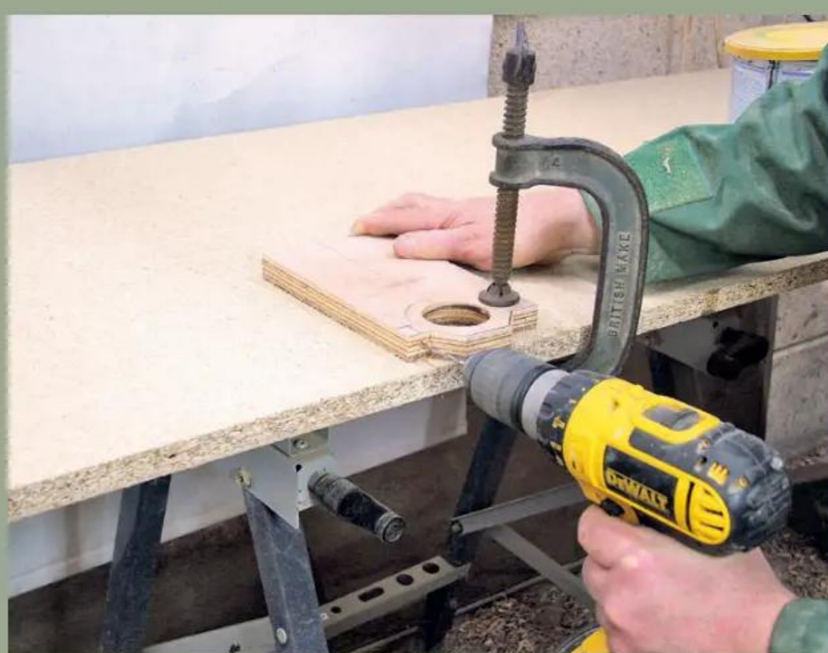
8 Drill pilot holes in the bracket, deep enough to run on into the upright
