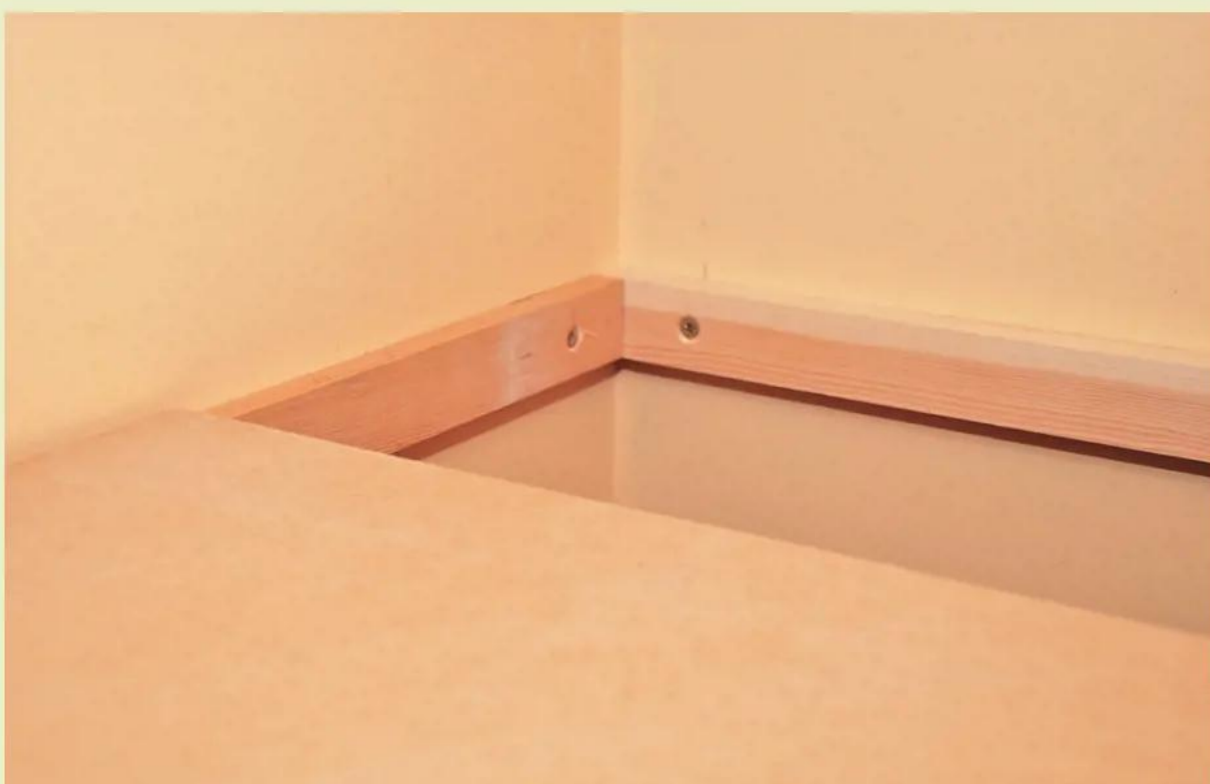
13 Fix battens to the alcove's rear and sides, checking they're level. Slide the shelf into place
