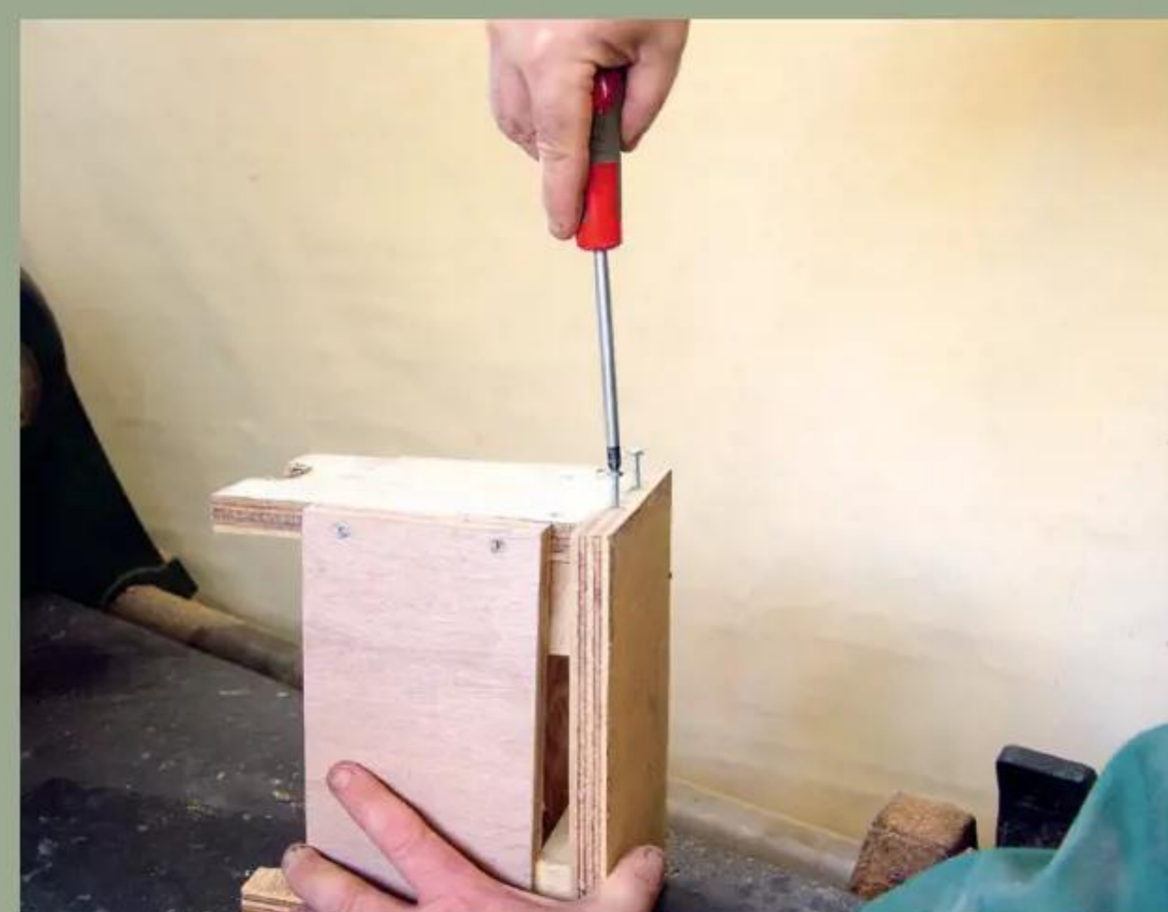
12 Drive two roundhead screws part-way into the cradle base's bottom edge
