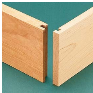
▲ A locking rabbet joint looks good, is fairly easy to make on the table saw, and provides a reasonable amount of strength.
