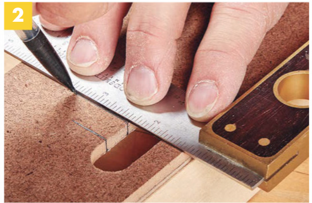
▲ Transfer Lines. Carry over the centerlines and marks from the paper pattern to the upper face of the jig. Marks inside the slot are used to align the workpiece.
