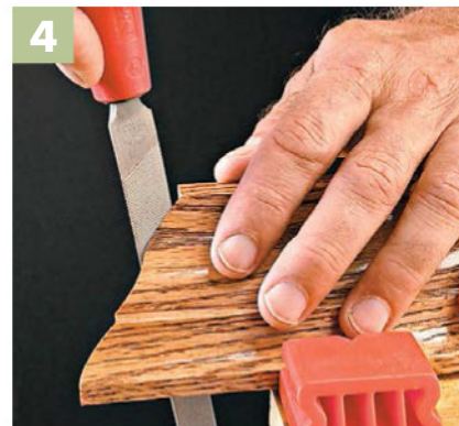
4 ▲ After completing the cope cuts, use a half-round file to refine the fit, working just up to the edge of the molding.
