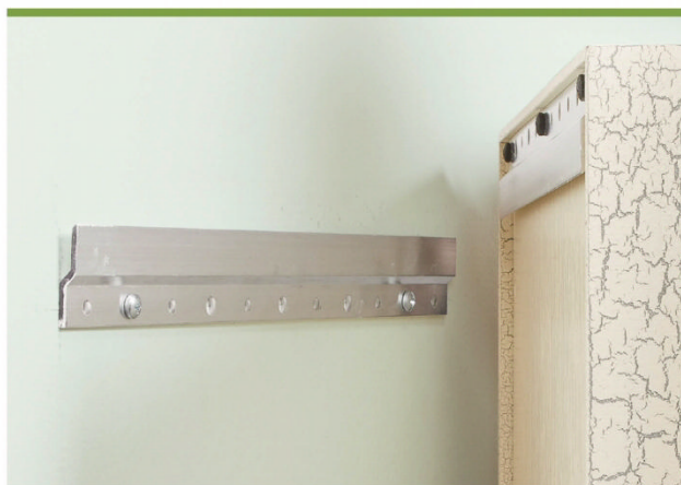
▲ The shadow boxes are mounted to the wall using a low profile, two-piece Z-hanger. This makes installation a breeze.
