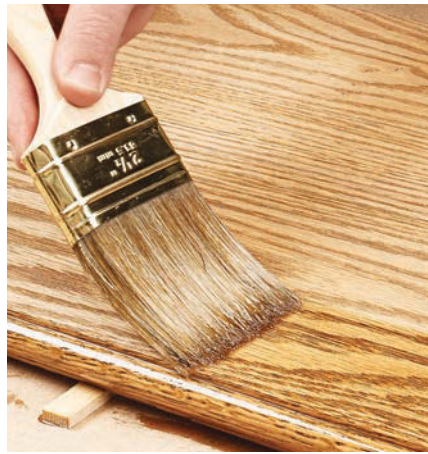
▲ Now move back to the starting point, and make a smooth, sweeping stroke with the grain across the panel.
