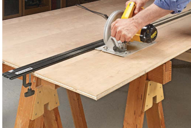
▲ When breaking down full sheets, be sure to use enough sawhorses so that the offcut and the main sheet are fully supported.
