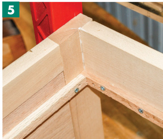
Supporting Strips. Pre-drill the ledger strips that will support the well bottom. Once these are in place, you can add the bottom for the top well of the box.
