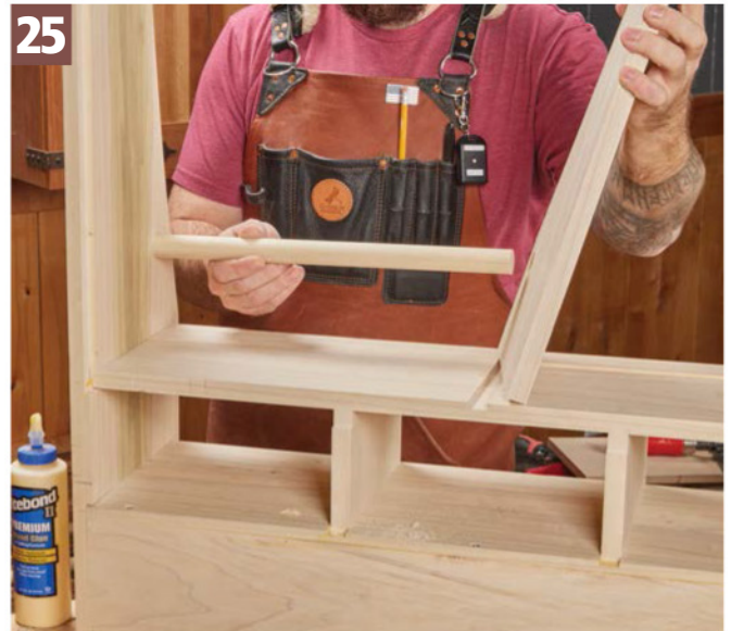
25 Tool Rest Glueup. Glue the dowel for the tool rest into place. In order to slip it in, you'll need to tip the saw divider as you insert it.
