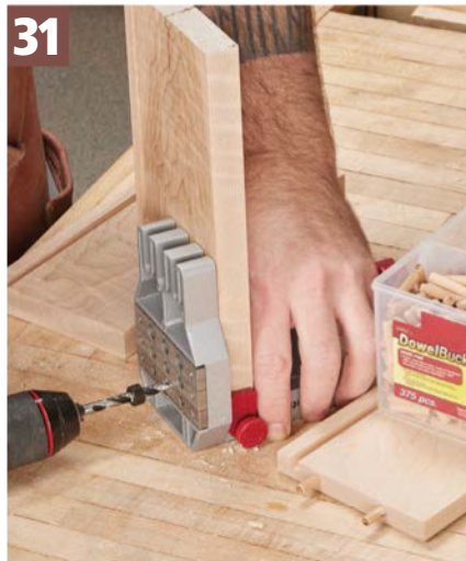
31 Dowel Holes. Drill the dowel holes in the edge of the sides, and faces of the fronts. I chose to use a doweling jig for these.
