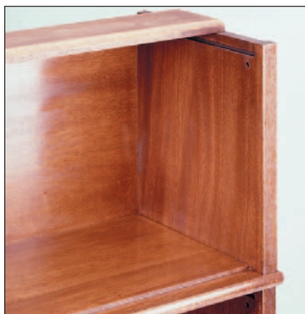
Since it's never really seen, there's no top to the bookcase — just a top cleat that interlocks with the two bottom cleats in the case section above it.
