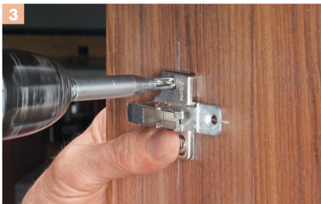
▲ A small piece of double-sided tape helps hold the plate in position while you drill pilot holes. While you want to do careful work, the hinge is easy to adjust so don't sweat it if you're off slightly.
