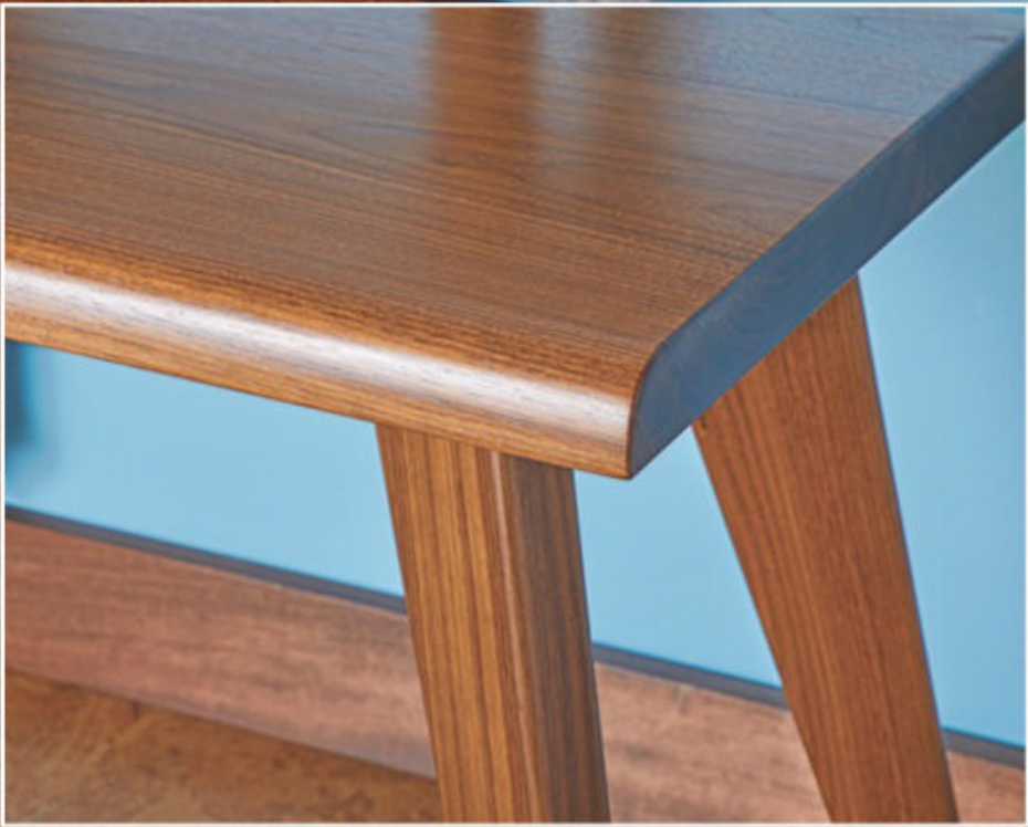
▲ The angled, tapered legs are up to the task of providing sound support for this bench. Also, the large roundover on the front edge guarantees it's a comfortable resting place.
