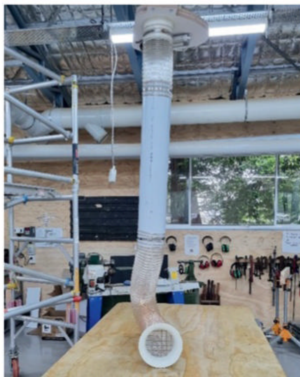
▲ Bell end bench sweep on the sanding bench. There is also a manually operated floor sweep.
