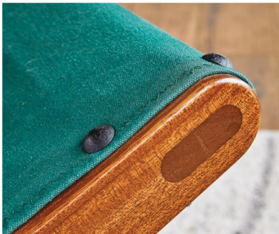
▲ The decorative nails used to hold the canvas sling in place are called clavos nails. Although they're decorative, they have plenty of strength to do the job required. The large, round heads add a nice accent to the chair.
