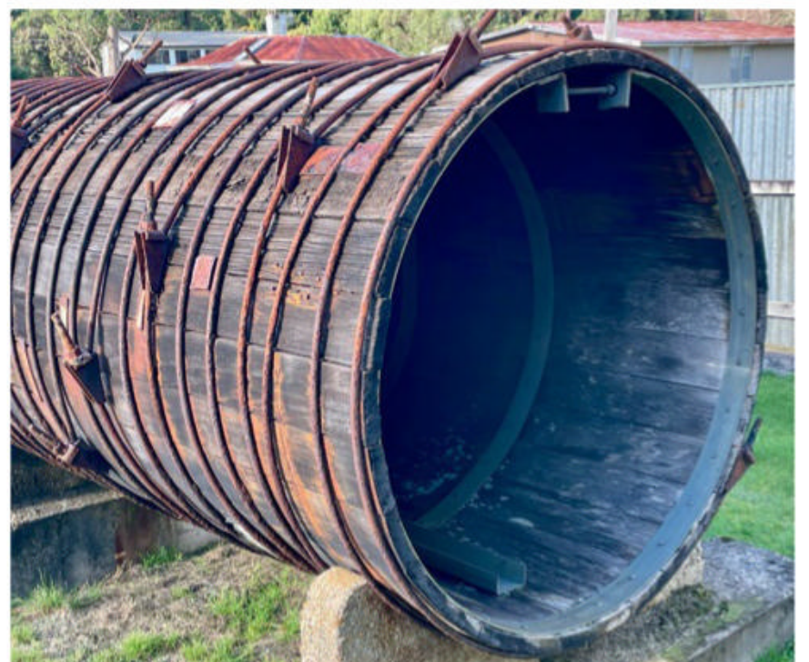
▲ This section of Lake Margaret penstock was originally made from Douglas fir. In 1938 it was rebuilt with King Billy pine staves.
