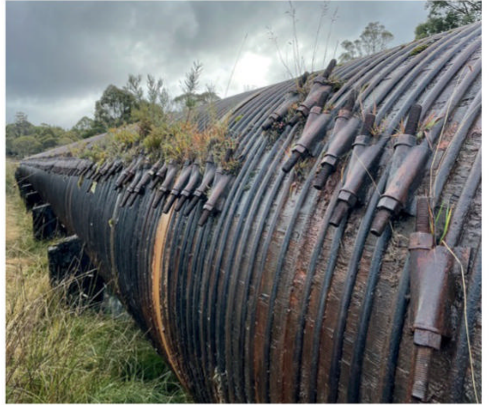
▲ The wooden penstock featured on these pages runs beside Laughing Jack Road, off the Lyell Highway, east of Derwent Bridge.
