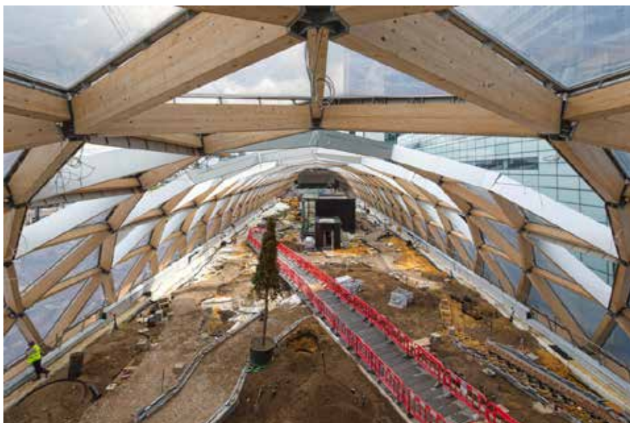
Photograph showing the first tree (a magnolia) is installed in the roof garden above canary wharf crossrail and the detail of the roof construction
