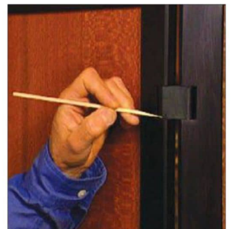
FIGURE 5 Installed in the hinge, the brass pins are inserted into the slots on either side of the notch in the frame. A spline is cut to size to fill the slot and hold the pins in place.
