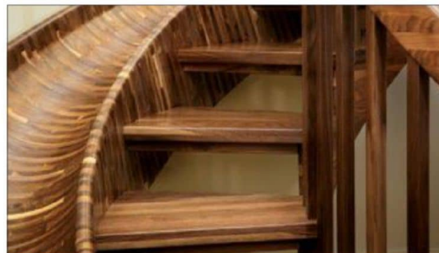
The laminates of the slide were cut on a CNC machine.
