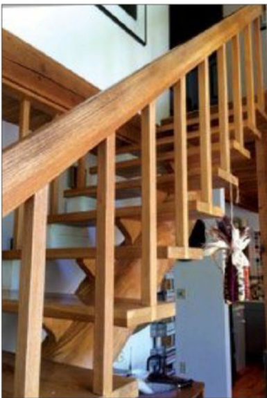
Jim constructed his home, mostly using milled trees grown on his property. The stairway is White Oak, with treads suspended by dovetail joinery.
