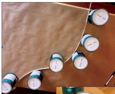
FIGURE 3. You will need to move cans out of the way to draw the curve. Support the strip with your hand, draw that section, and move the can back.
