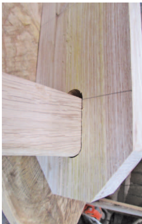
11 Fitting the key to the poppet mortice
