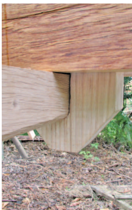
16 Hammering in the key to secure the poppet to the bed
