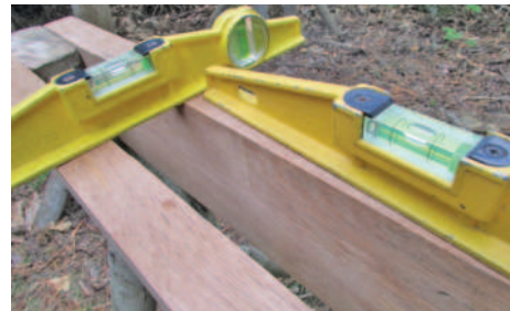
4 Checking the bed is level in both planes
